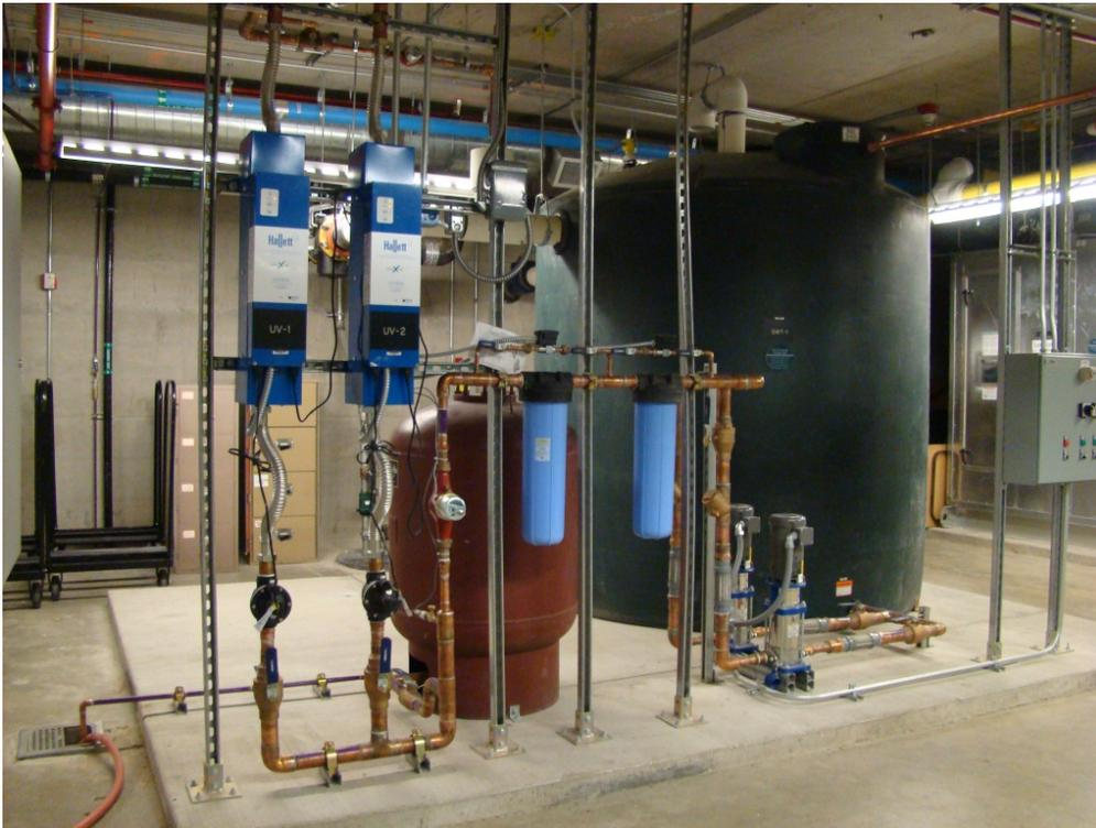
*Internal cistern stormwater collection tank at the Platinum LEED certified Tahoe Environmental Research Center (TERC) in Incline Village. Photo Courtesy of TERC.*
