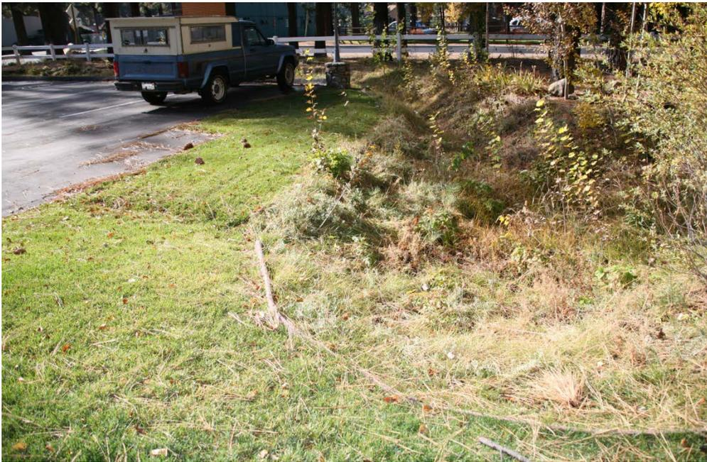
*A grass swale leading runoff from a small commercial parking area into a rain garden.*
