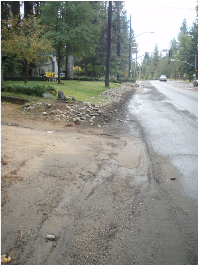
Sediment laden runoff entering the right of way from an unpaved driveway.
