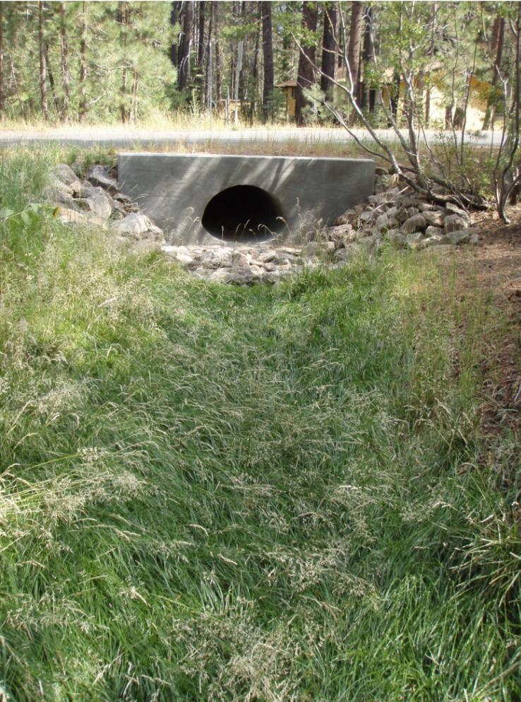
*Culvert conveying stormwater under a road and discharging to a vegetated swale.*
