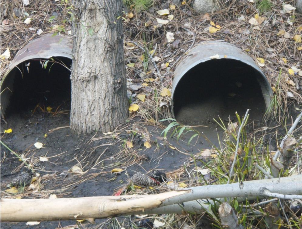
*The sediment at this storm drain discharge is a result of lack of maintenance within the drainage system.*
