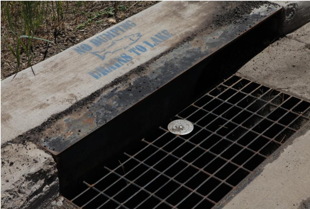
*Storm drain inlet conveys water to a subsurface storm drain.*
