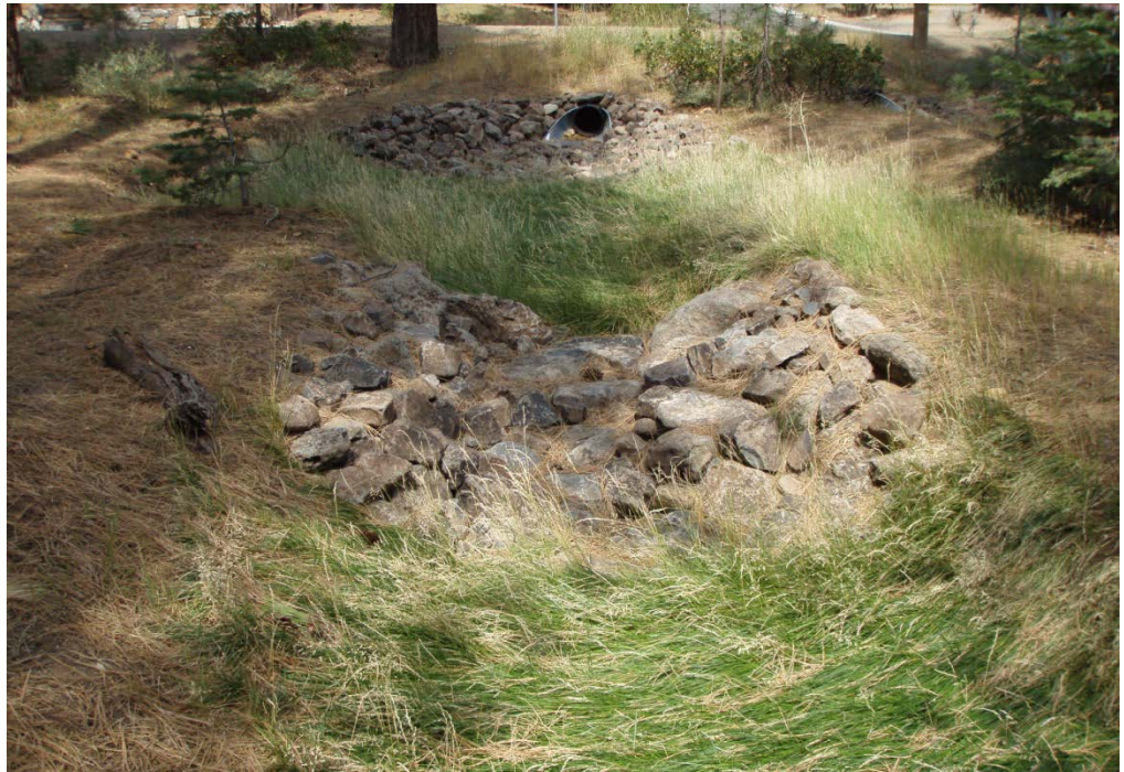
Check dams installed in water spreading area (top) and vegetated swale (bottom).
