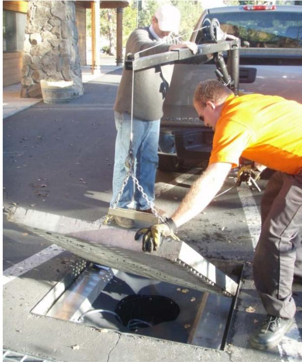
*Installation of a drop inlet insert for a commercial parking lot.*
