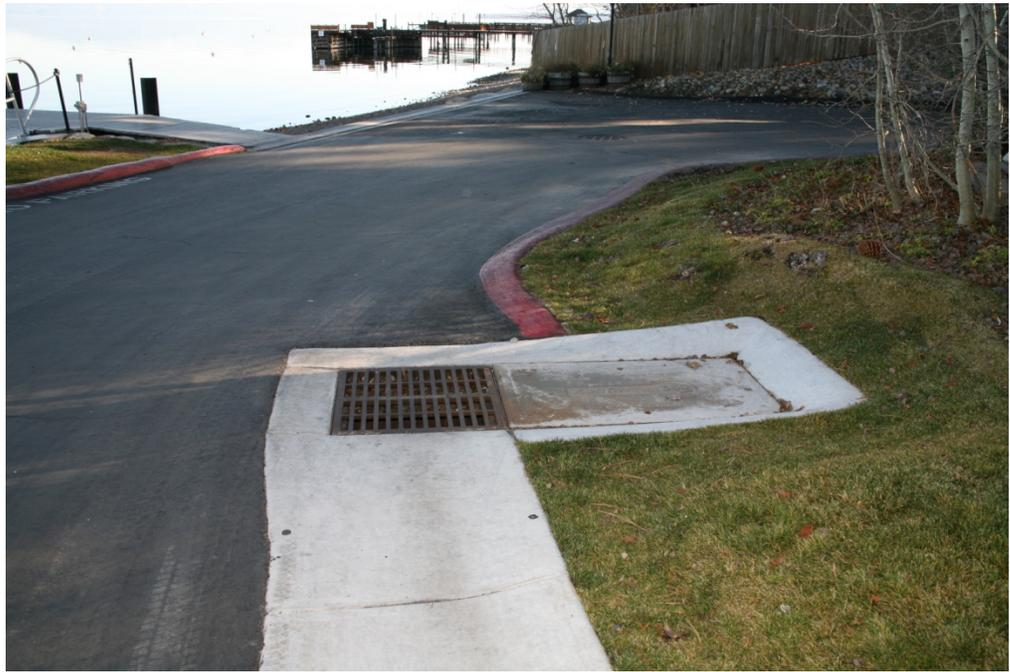
*A media filter installed on a commercial parking lot directly adjacent to Lake Tahoe to meet regulatory discharge standards where infiltration is limited due to high groundwater.*
