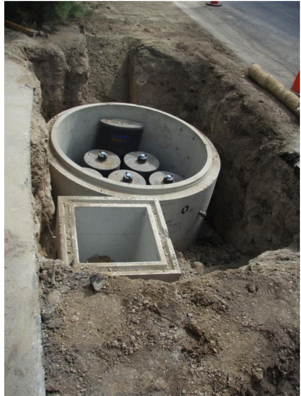
*Cartridge based filter installed at a commercial site.*
