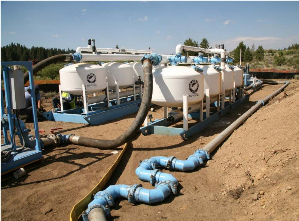
*A tank filtration and settling system set up to dewater groundwater for excavation work near the Upper Truckee River.*
