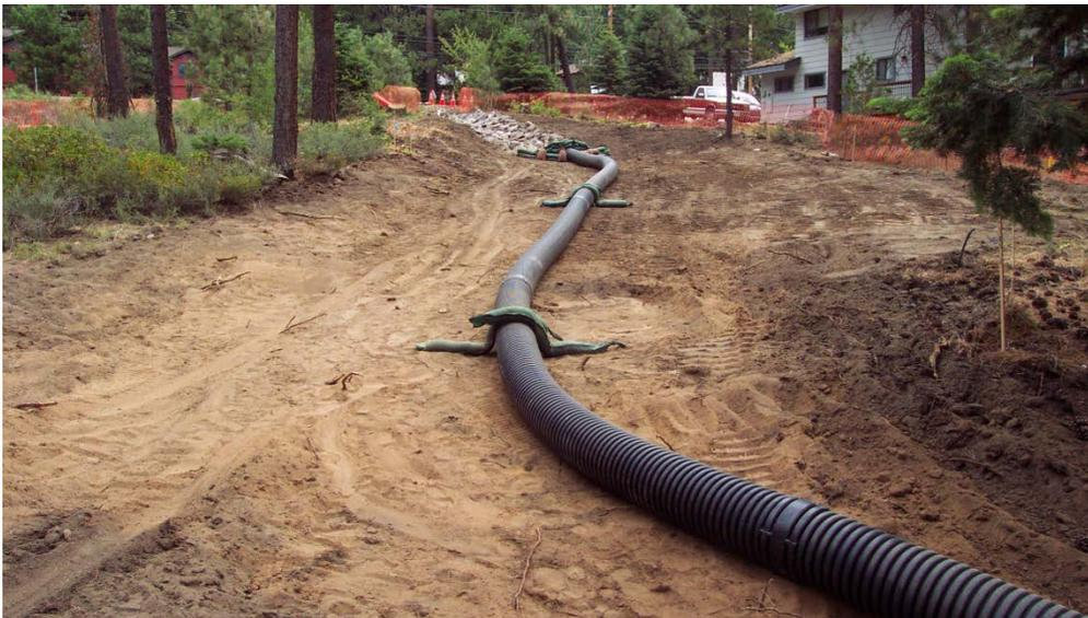
*Flexible downdrain diverting upstream runoff through a construction site during installation of BMPs.*
