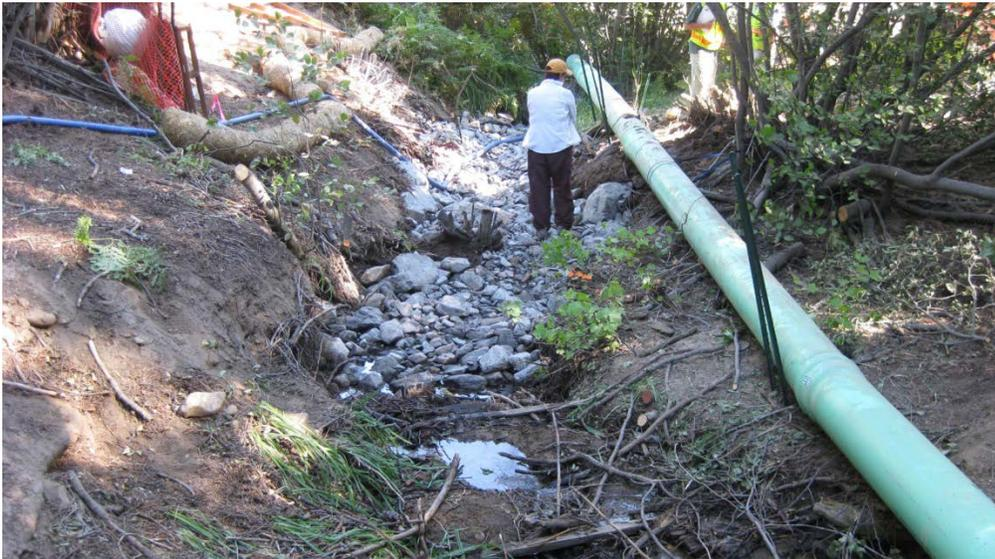
*Clean water diversion isolating a section of stream for project work.*
