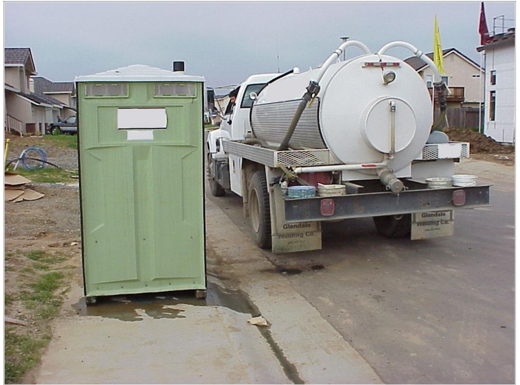
Improperly managed and leaking temporary sanitation facility.
