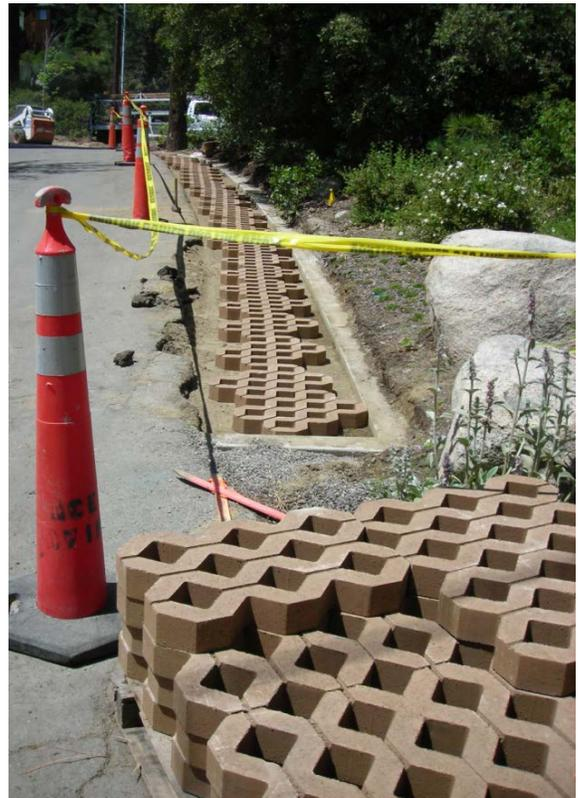
*Installation of open-celled pavers that will be filled with washed gravel on the edge of a narrow roadway in Crystal Bay.*
