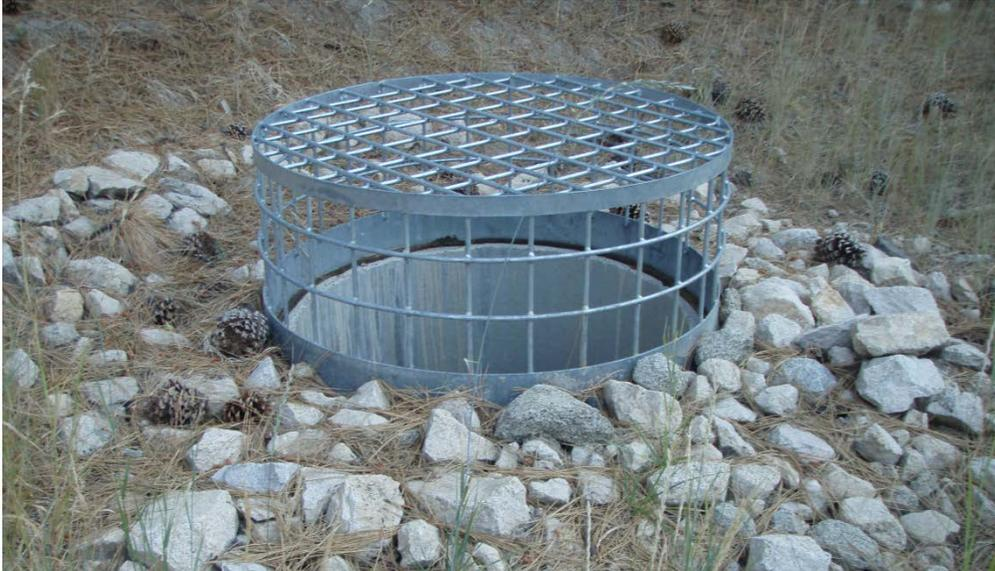
*This trash rack will prevent trash from entering the stand pipe in the basin.*
