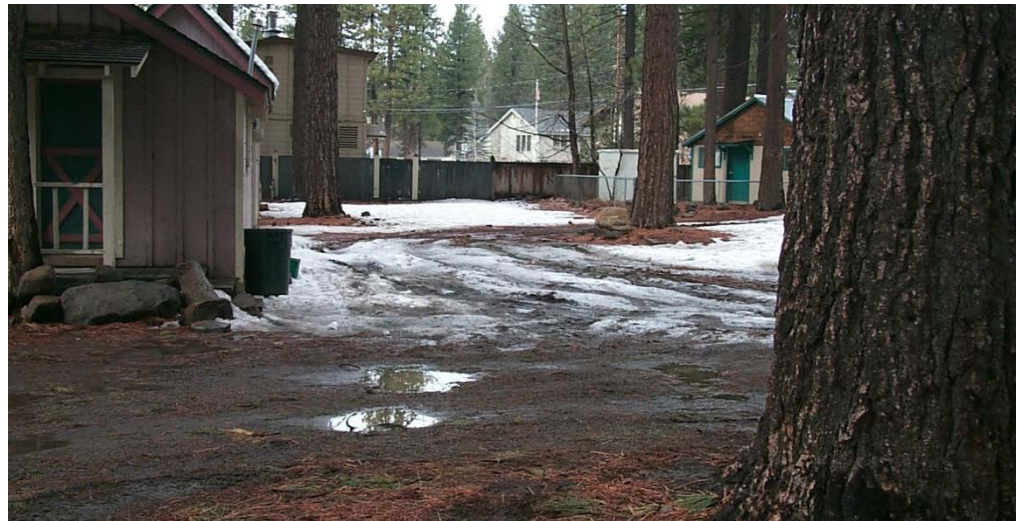
This unpaved driveway should be paved. It is currently a sediment source when vehicles track dirt onto the roadway and during disturbance from snow plows.
