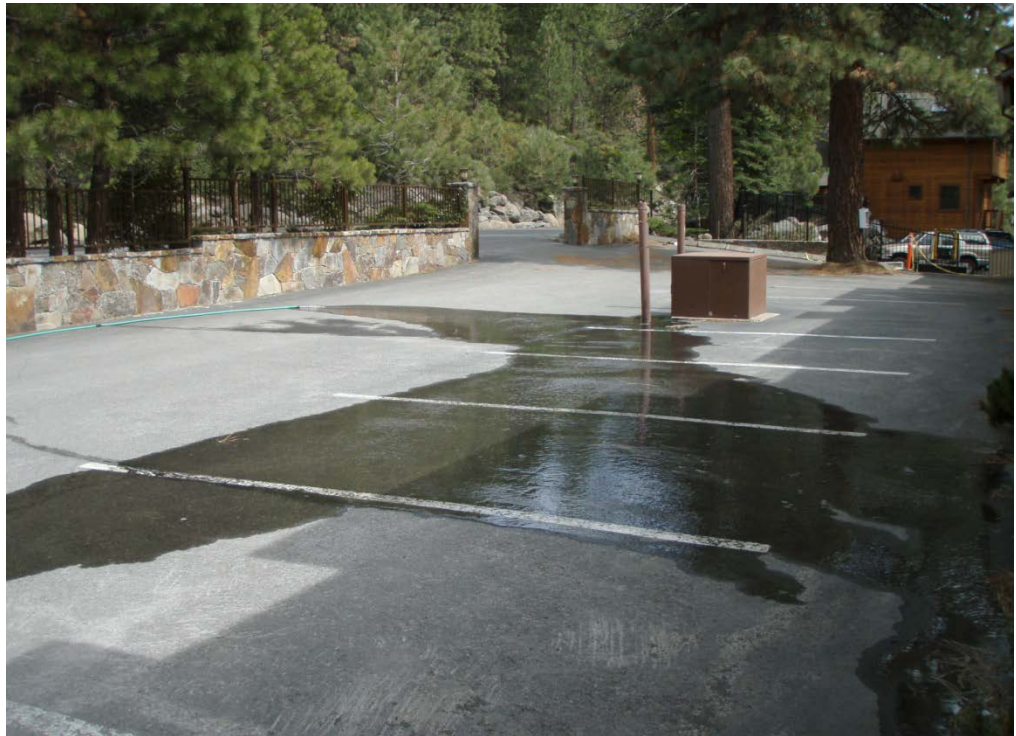
Running a hose on a property will help identify flow patterns on-site and can simulate what happens during a stormwater runoff event.
