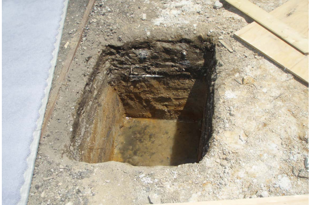
Soil pit dug in preparation for a soils/hydrologic investigation to determine the depth of seasonal high ground water.
