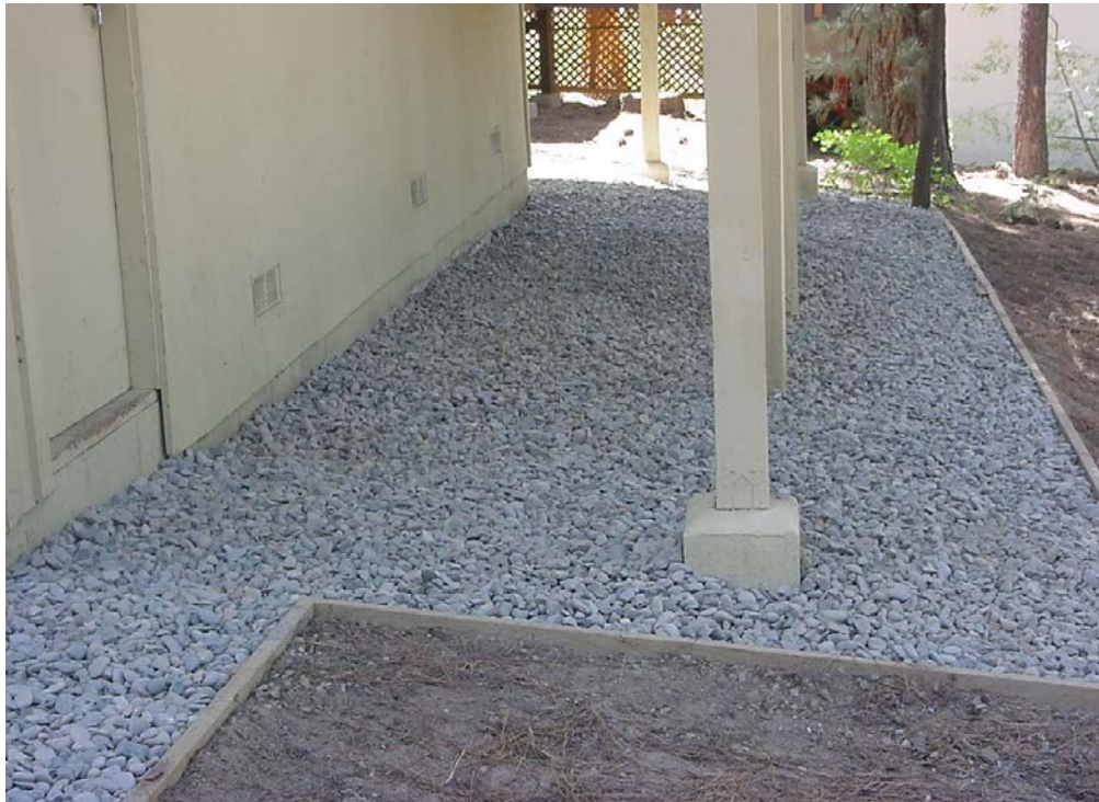
This deck has 3 inches of gravel underneath and is bordered with lumber that is treated to be fire resistant.
