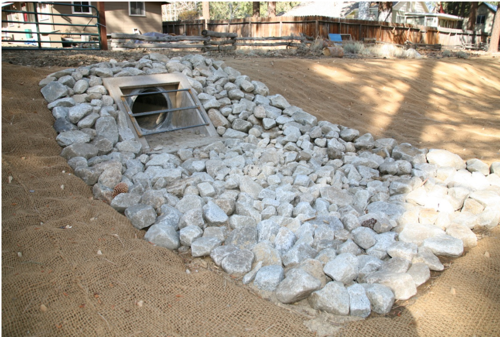
Recently constructed rock outlet protection
