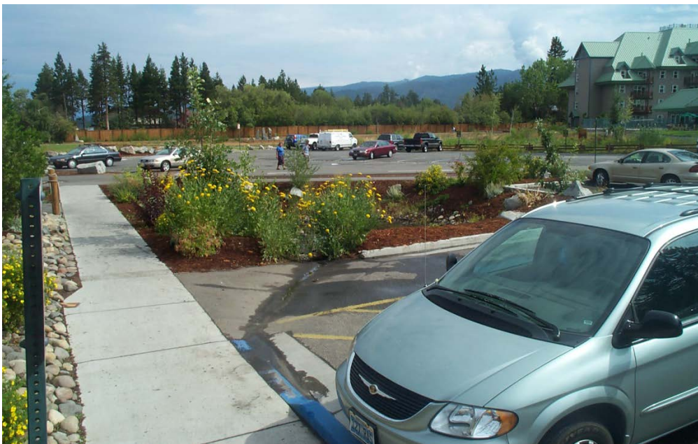
A small landscaped rain garden captures and infiltrates stormwater runoff from a Lake Tahoe marina parking lot.
