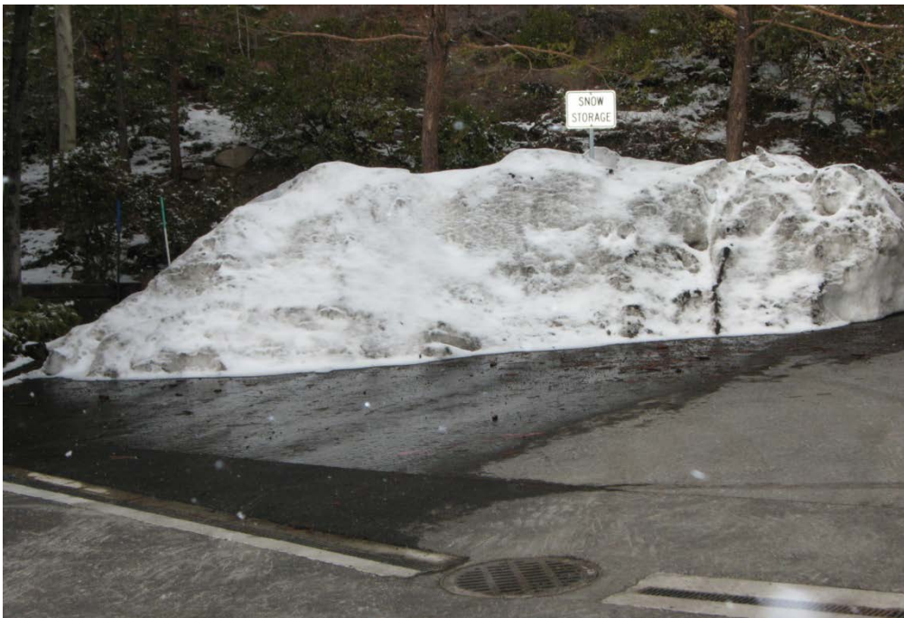
This snow storage area is ideal because it is on a paved surface, upslope of drainage BMPs and the sign clearly indicates the area is dedicated for snow storage.
