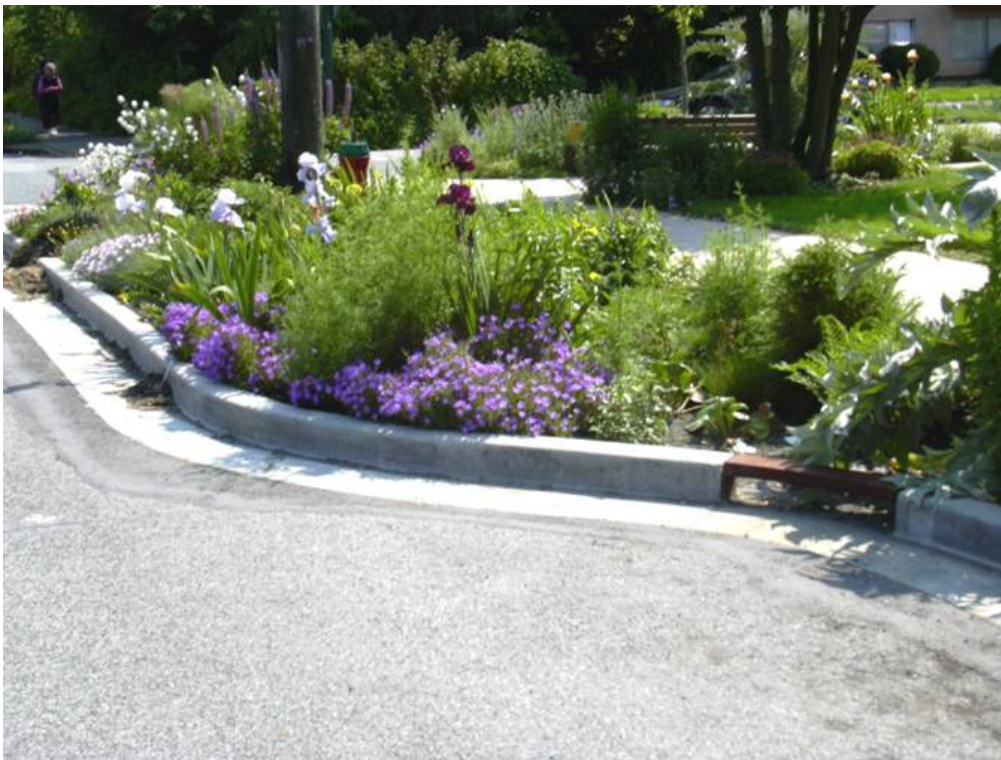
This curb cut breaks up concentrated stormwater and discharges to a vegetated depression.
