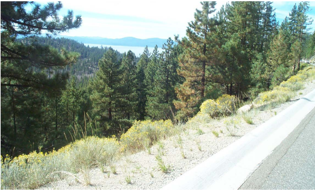
Curbs convey clean stormwater from a road, preventing it from discharging down the steep slope, potentially causing erosion.
